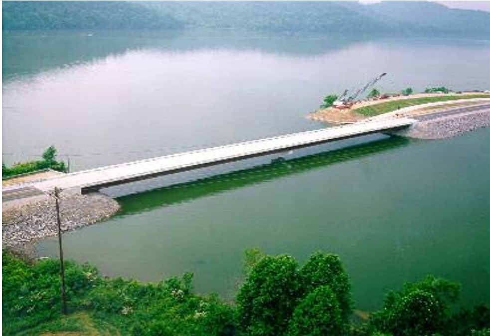
Figure 1. State Route 53 over Martin Creek
