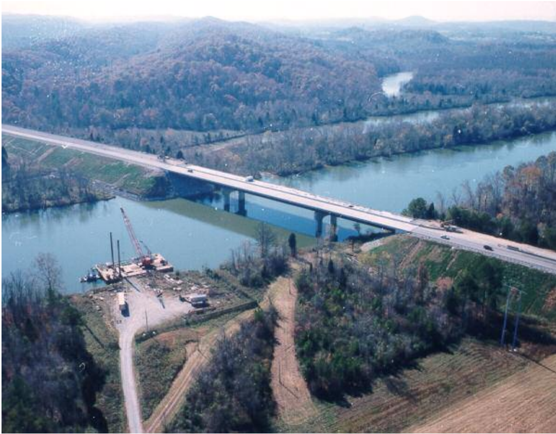
Figure 3. State Route 58 over the Clinch River
