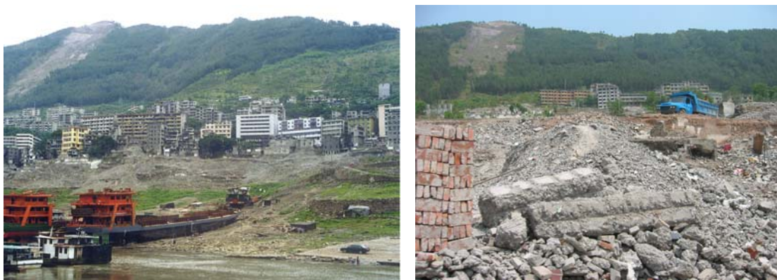
Figure 2. Yunyang, a county town, is threatened by a landslide in the rear part and to be inundated in the front part. By 2005, much of the town was demolished
